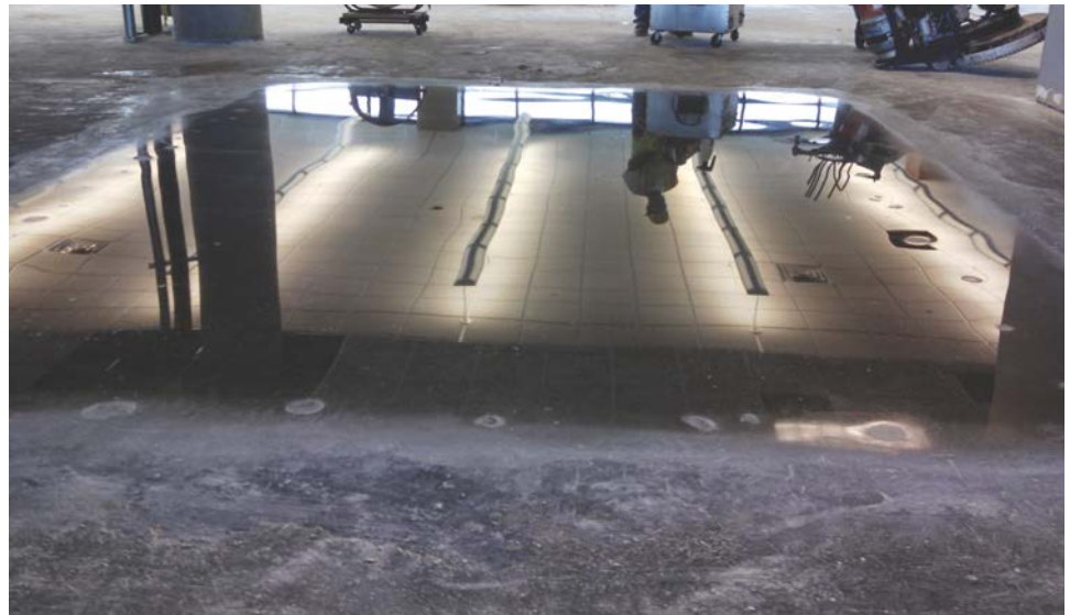
This concrete floor test panel in an under-construction Minneapolis-based corporate headquarters displays a roughness average of 2 µin (microrinches), or an A-1 surface texture grade, the highest level of refinement on the ST 115 surface texture finishes chart. Photo courtesy of Ryan Companies of Minneapolis.
