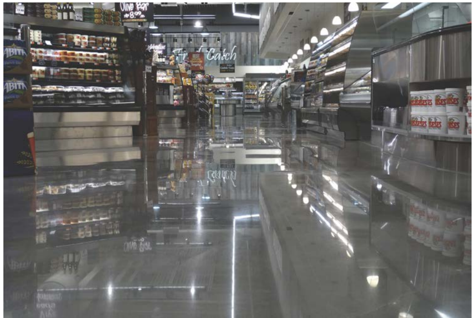
Measured for roughness average after every pass of grinder and polisher, this concrete floor in a high-end New Orleans grocery store shows an ST-115 A-2 finish, equivalent to 5,000 grit. Photo courtesy of Prep and Polish Consultants LLC Dallas, Texas.
