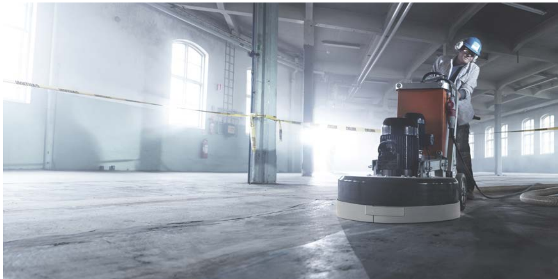
Measured for roughness average after every pass of grinder and polisher, this concrete floor in a high-end New Orleans grocery store shows an ST-115 A-2 finish, equivalent to 5,000 grit. Photo courtesy of Prep and Polish Consultants LLC Dallas, Texas.
